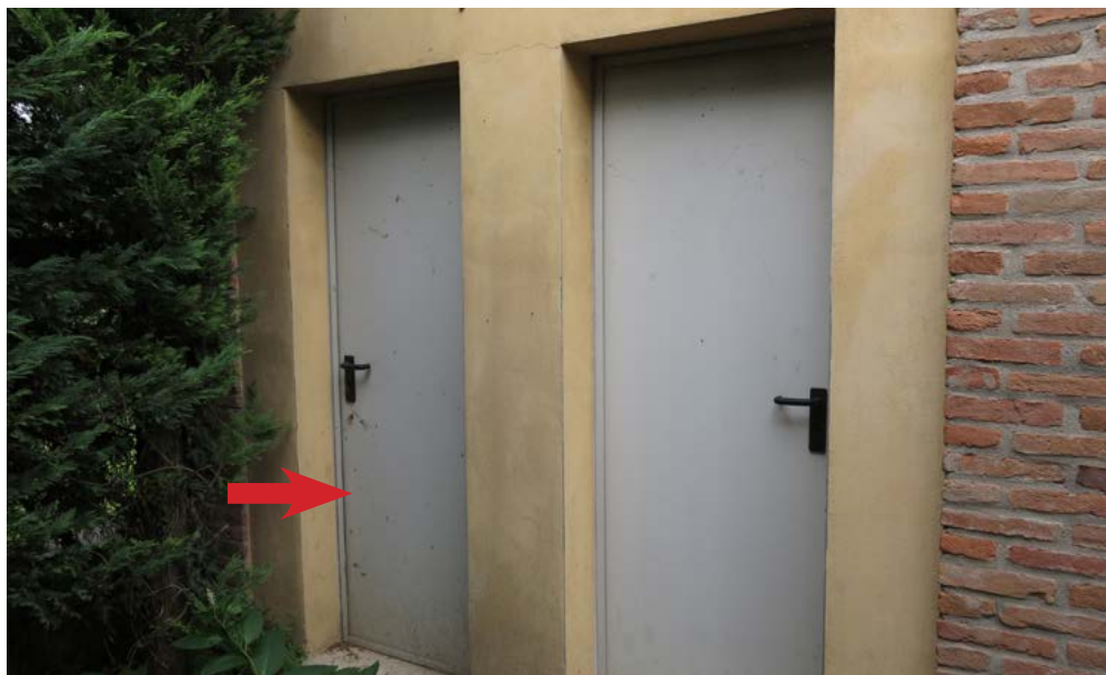
Cantina, piano terra lotto 13.
