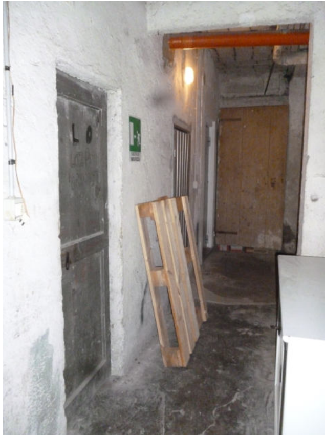
FOTO 15 – Piano S, area cantine
